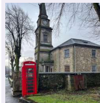
Lochwinnoch Parish Church Owned by LCDT and in process of being upgraded as a community facility.
