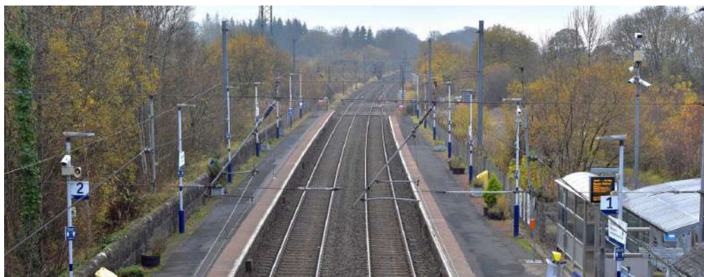
Figure MA0a | Lochwinnoch Rail Station
