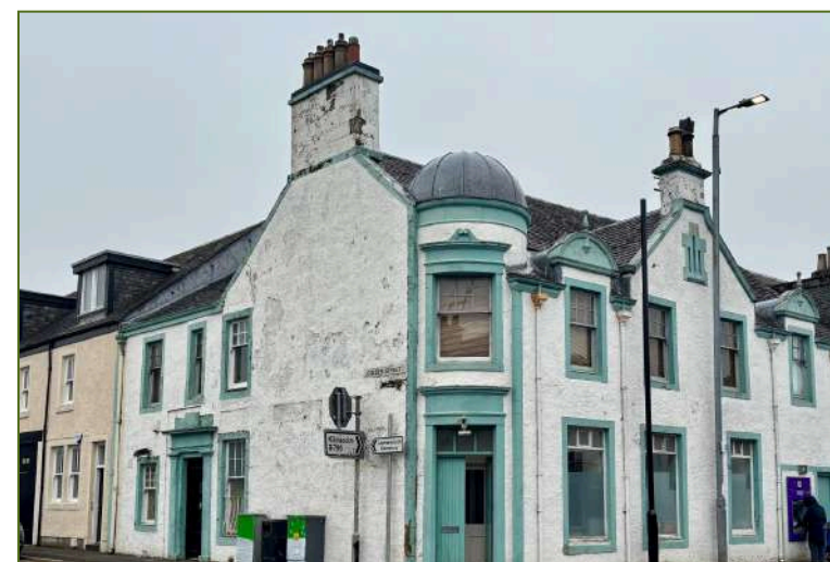
Figure PS1b | Old Bank building, Lochwinnoch highstreet (credit: LCDDT)
