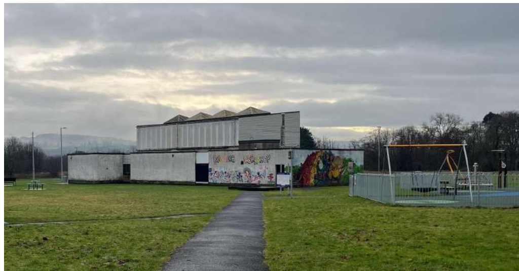
Figure F0b | The Annex and public playpark
