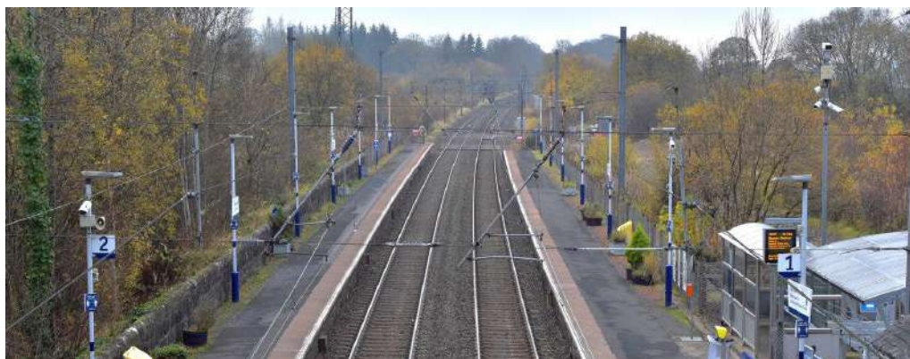
Figure MA0a | Lochwinnoch Rail Station
